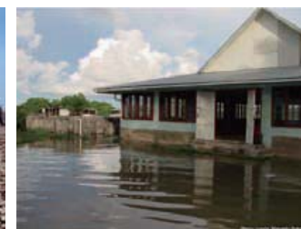
Damage caused by sea level rise (Funafuti island, Tuvalu)
